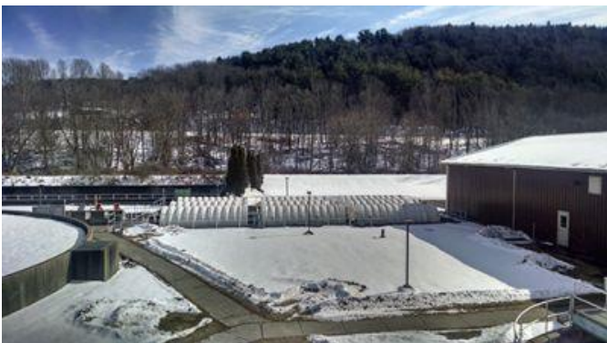
Rotating Biological Contractors
